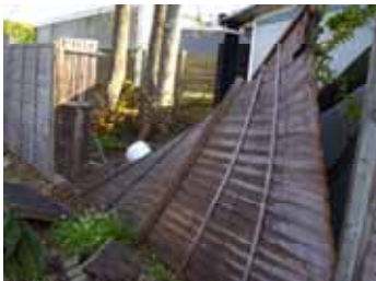
< Final Lap A poorly erected structure combined with an exposed position reduces the life of a wooden boundary fence.
