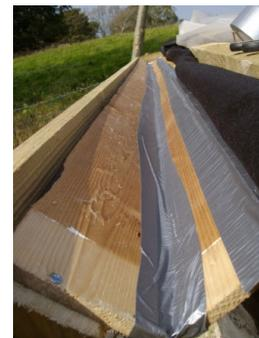
9. Use strong duct tape to seal the edges of the slats to the OSB board and bottom of the joint. Add downpipe.
