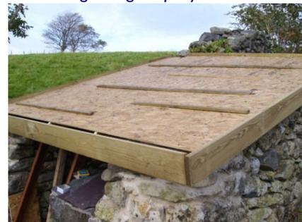
3. As the roof pitch is quite high, I fixed battens to the boarding to prevent the plant material from slumping. These battens will also catch and slow down the flow of rainwater.
