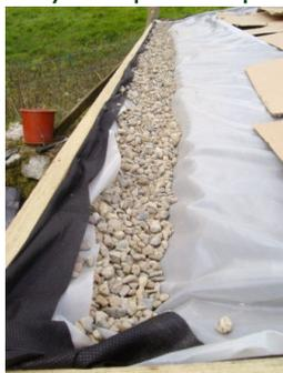
10. Fold underlay and polythene into gutter and staple neatly to top of lower cladding timber. Fill with pea shingle.
