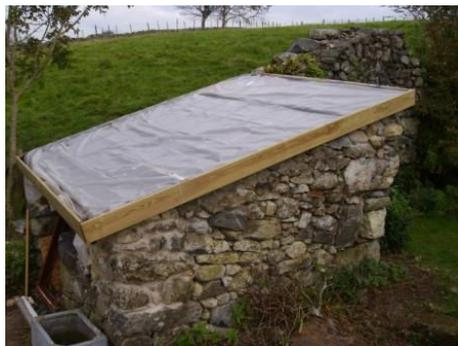
7. Cover with heavy duty polythene, loosely over the battens and staple a seam with the underlay to top of 2" 'lip'.
