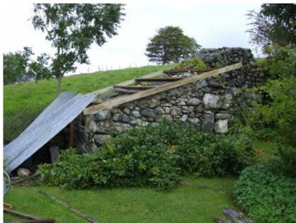
1. I used 3"x3" posts and 4"x1" cladding, fixed to the ends of the posts. The posts were firmly secured to the top of the stone walls with lime mortaring
