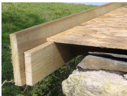
4. Fix 6"x1" cladding to the existing cladding timber. This will give you a 2" lip for soil and plant materials.
