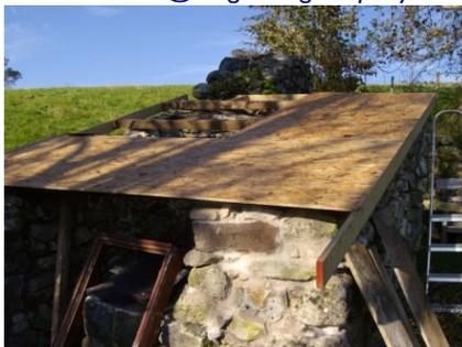
2. Fix exterior grade OSB (Stirling) Board to the posts and cladding timber. Note the timber cladding extends beyond lower pigsty front.
