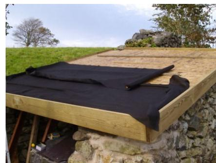
6. Cover board and battens with underlay and staple. Allow enough material to overhang edges.
