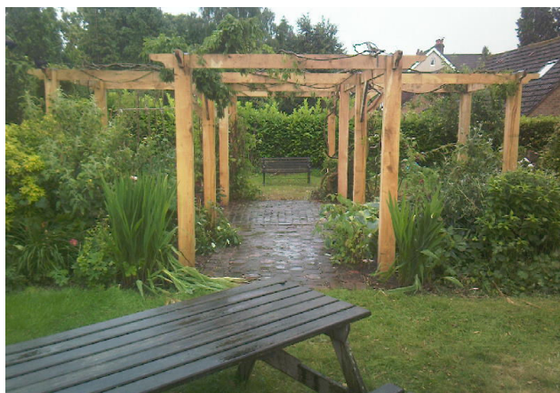
v> AFTER: the decision was taken to demolish the brick pillars and completely rebuild the pergola frame in oak, in a new, larger cruciform shape
