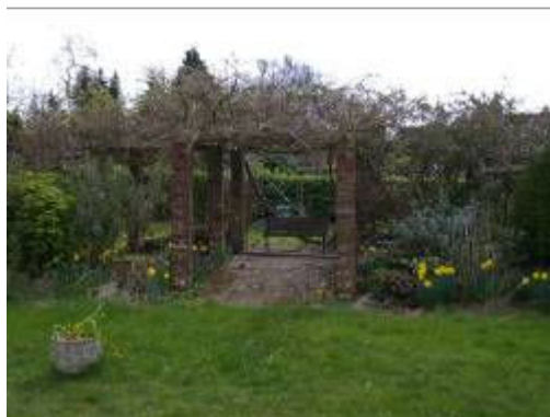
< ^ BEFORE: This half-century old brick pillar pergola is slowly being crushed by the weight of the mature Wisteria
