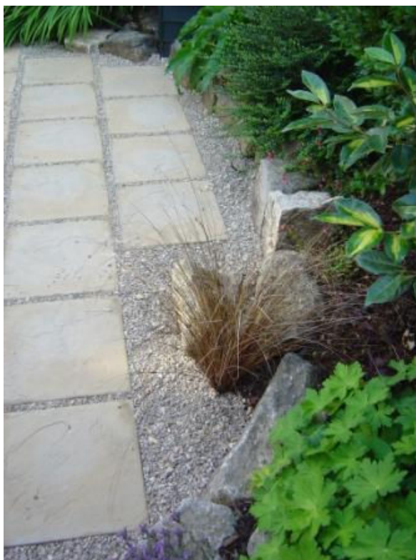
^ v AFTER: slabs laid in rows at an offset angle with wide gaps between slab rows filled with fine shingle
